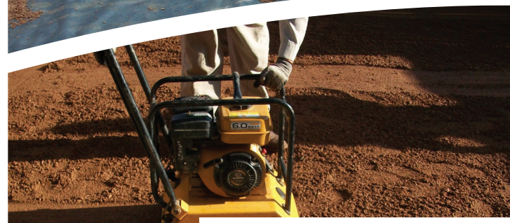
Sub Base Compaction
